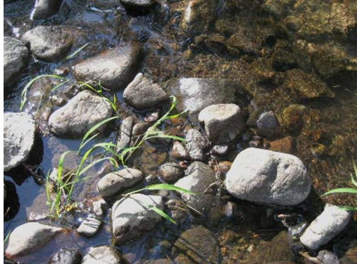
Photo 7-1. Void-filled riprap is designed to emulate natural rock riffle material and able to support riparian vegetation (Mile High Flood District, latest edition)
